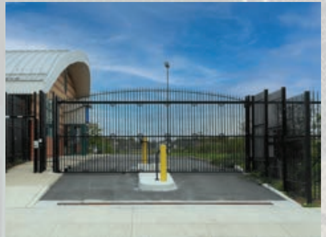
Right: Structural Cantilever Slide Gate.
