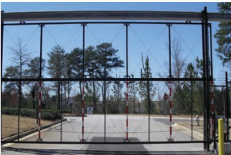
Right: Overhead Slide Gate.
