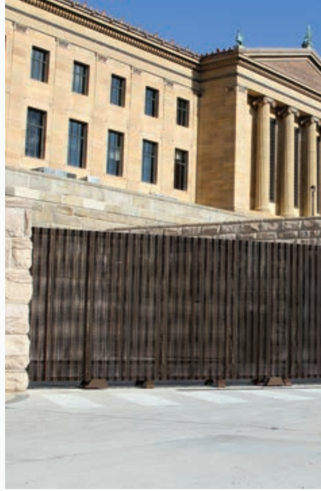
Right: Box Frame Roller Gate, Clear opening width 60 feet 2 inches by 10 feet high, Pg. 18
