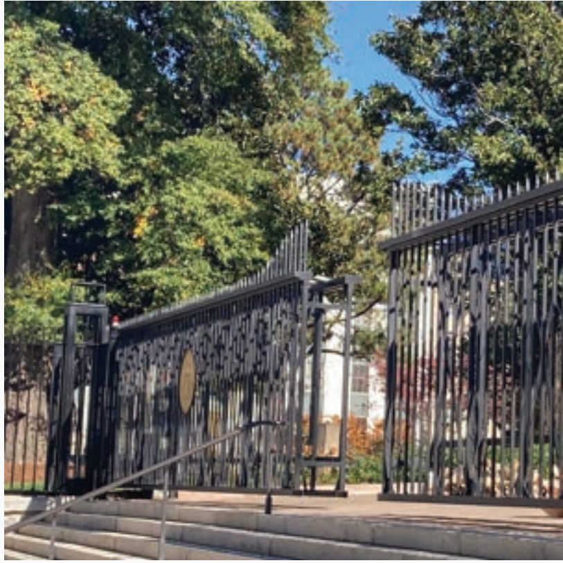
Right: Bi-Parting Box Frame Cantilever Gate with an opening of 61 feet. Pg. 15 for more details.
