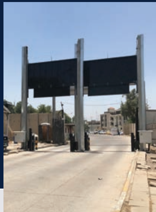
Right: Green Zone, Iraq, K12 Rated Vertical Lift Gates.
