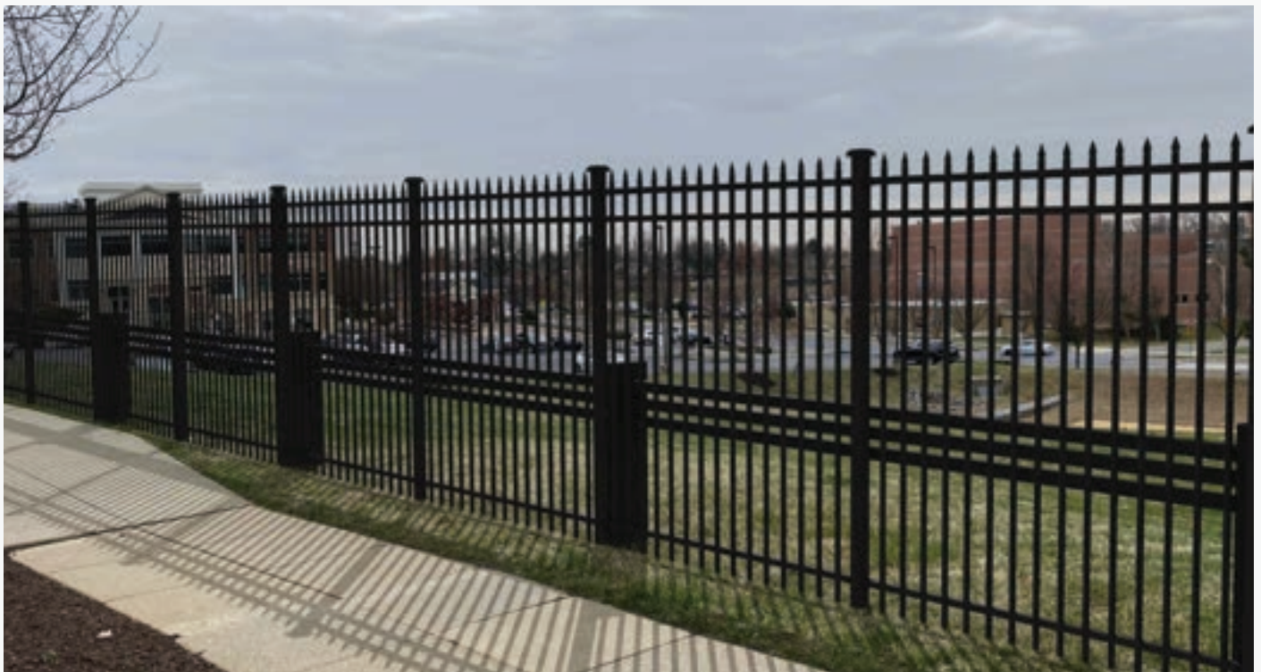
Right: TCF Crash Cable Barrier.
