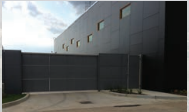
Right: Structural Cantilever Gate.
