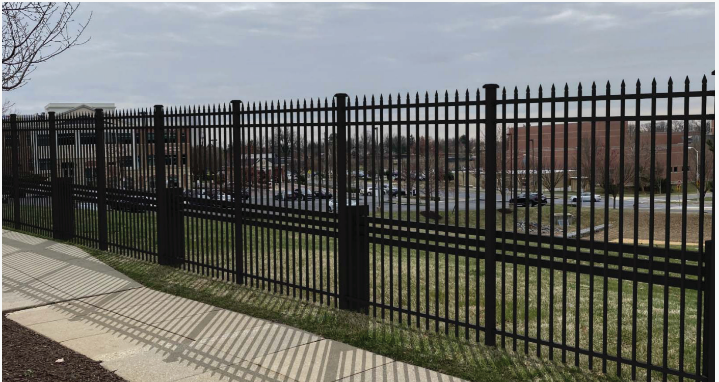
Right: TCF Crash Cable Barrier.
