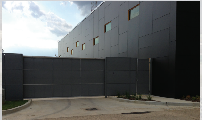
Right: Structural Cantilever Gate.
