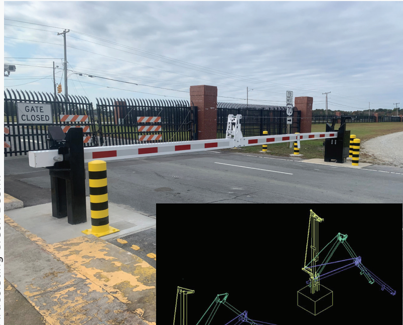
Right: Cherry Point Marine Base, ATCRB-12 Articulating Crash Beam.
